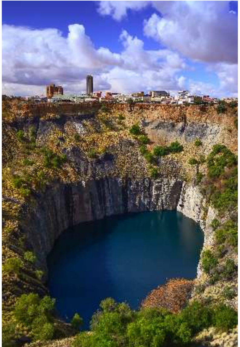
Above: The Kimberly Mine (aka 'The Big Hole'). From mid-July 1871 to 1914, 50,000 miners dug the hole with picks and shovels, yielding 2,722 kg of diamonds.
